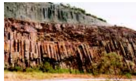
Columnar jointing occurs at the bottom of the rock face at the NE end of the dam. This is overlain by subhorizontal patterns, with shotcrete covering vertical joints at the top.
